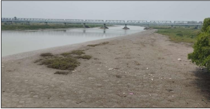
Fig. 5A- Photo of Waterspread Area near Advihal Bridge
