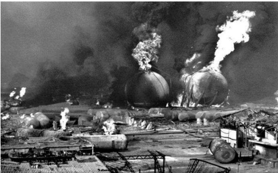
Figure 2: Boiling liquid expanding vapour explosions (BLEVE's) triggered by earlier vapour cloud explosions (VCEs) at Feyzin (France) (accidentsoilandgas.blogspot.in), top and San Juan (Mexico), bottom (devastatingdisasters.com/san-juanico-1984/).
