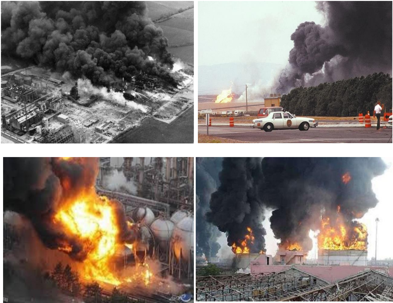
Figure 3: Damage caused by vapour cloud explosion at Flixborough (top left) ( devastatingdisasters.com/san-juanico-1984/ ), PEPCON (top right) ( damninteresting.com/the-pepcon-disaster/ ), BP refinery (bottom left) and Jaipur (bottom right) ( nbcnews.com/id/33800042/ns/world_news ).
