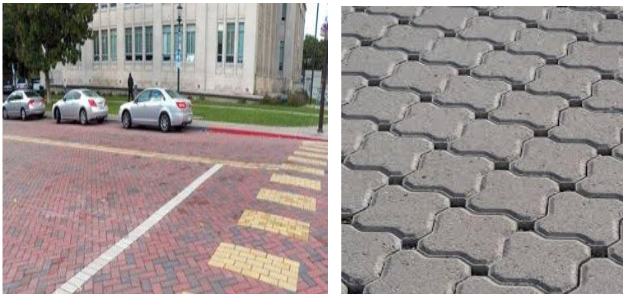
Figure 1.2: Typical Interlocking Concrete Pavements
