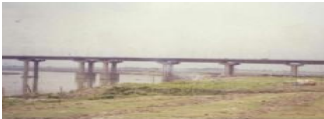
Fig. 1.2 Bridge on river Ganga at Allahabad having circular compound bridge pier
