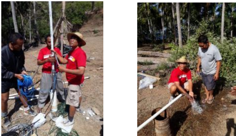
Figure 14. Pump Installation in Drilling Well
