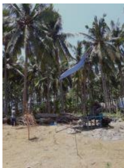
Figure 13. Drilling on Line Measurement 3 Point 99.75 m
